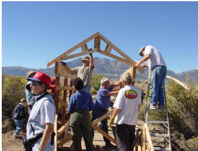
Marysville Kiosk construction. Photo courtesy of Max Reid.
